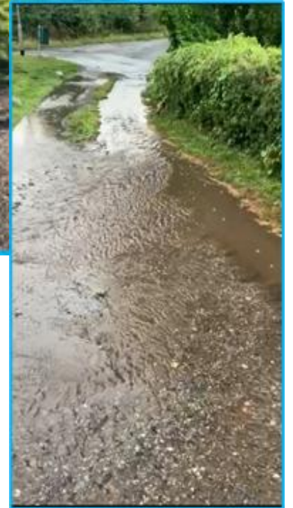
Brewood , South Staffordshire, Chillington Brook and surface water flood risk issues
